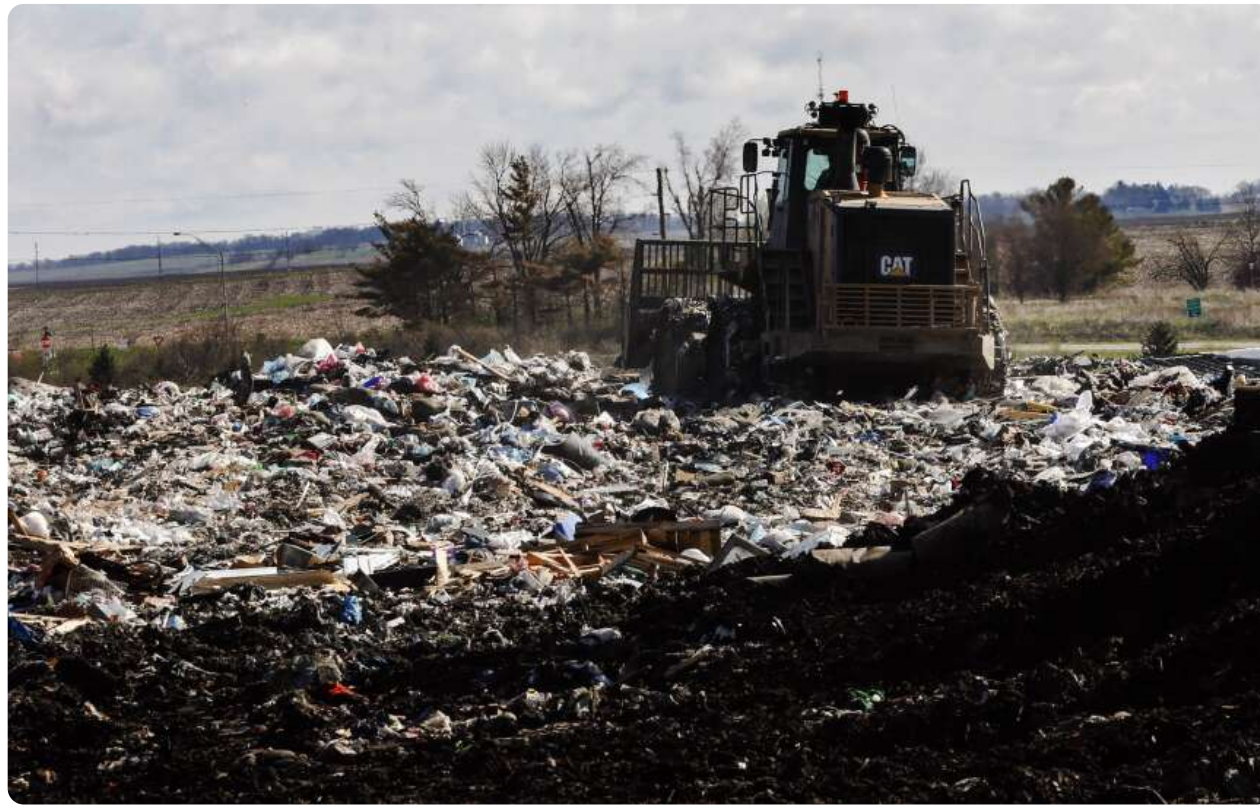
A bulldozer spreads and compacts refuse in May at the top of the current landfill cell at the Cedar Rapids Linn County Solid Waste Agency recycling and landfill site, 1954 County Home Rd., in Marion. (Jim Slosiarek/The Gazette)
