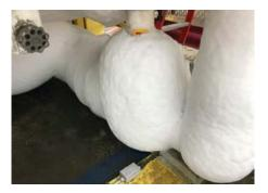
Insulation is a component of the refrigeration system. If it is displaced by ice, then it is not compliant with IIAR6, Section 5.6.8.2.
