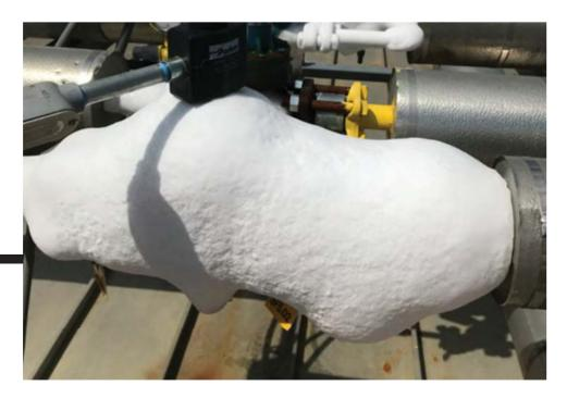
But what about a more significant amount of ice buildup on a valve train? Say, perhaps what is evident in the picture on the top right?
