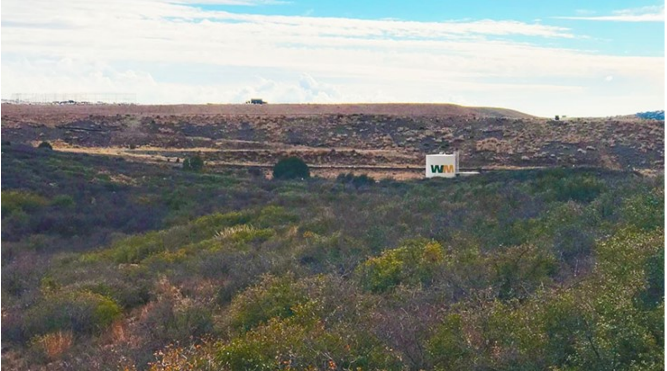
Photo courtesy of SCS Engineers
