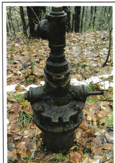
This unplugged well is leaking oil. Other abandoned or orphaned wells pose less obvious but equally unwelcome risks. Fortunately, cleaning up wells is becoming easier thanks to funding from government agencies and private organizations.
