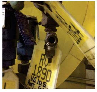
As operators get pressed for time, they often overlook final steps in operating procedures, such as reinstalling plugs on drain valves.
