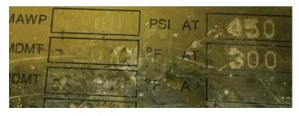
Often, it is not operators that lack attention to detail, including applicable codes and standards. The transfer drum below was installed on a -45°F recirculator. Note, that it is not dual rated and its Minimum Design Metal Temperature is -20°F.
