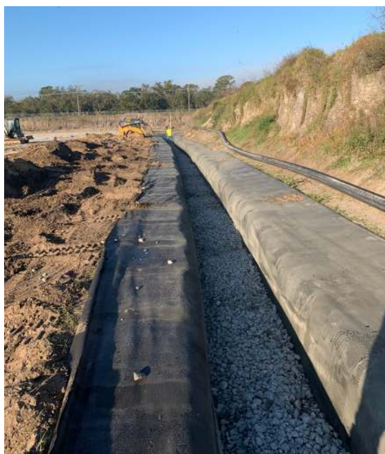
Figure 2 - Early collector installation at the Lena Road Landfill.
