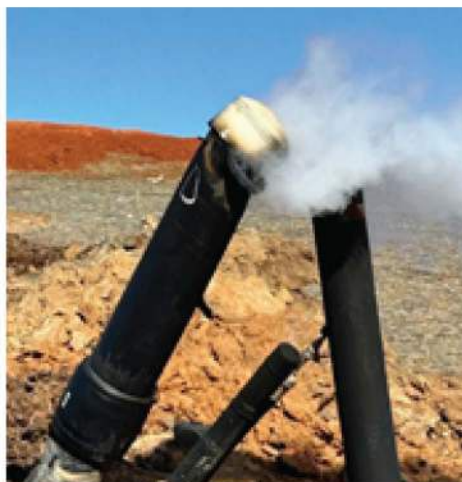
Figure 2 - Subsurface fire due to compromised infrastructure.
