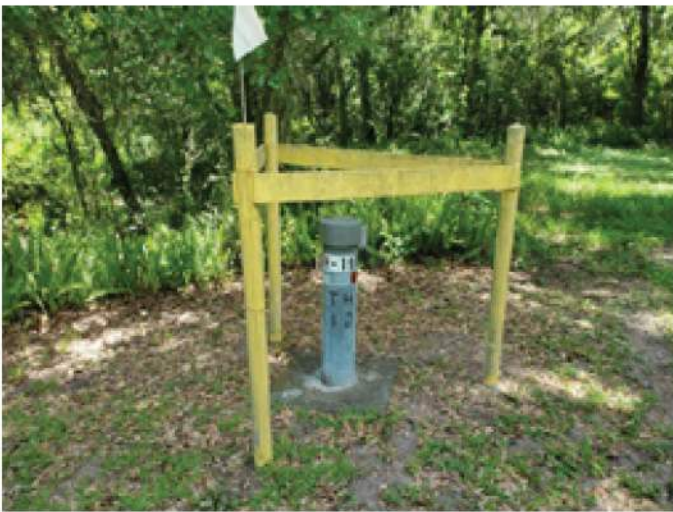
Typical groundwater monitoring well at a Florida landfill.
