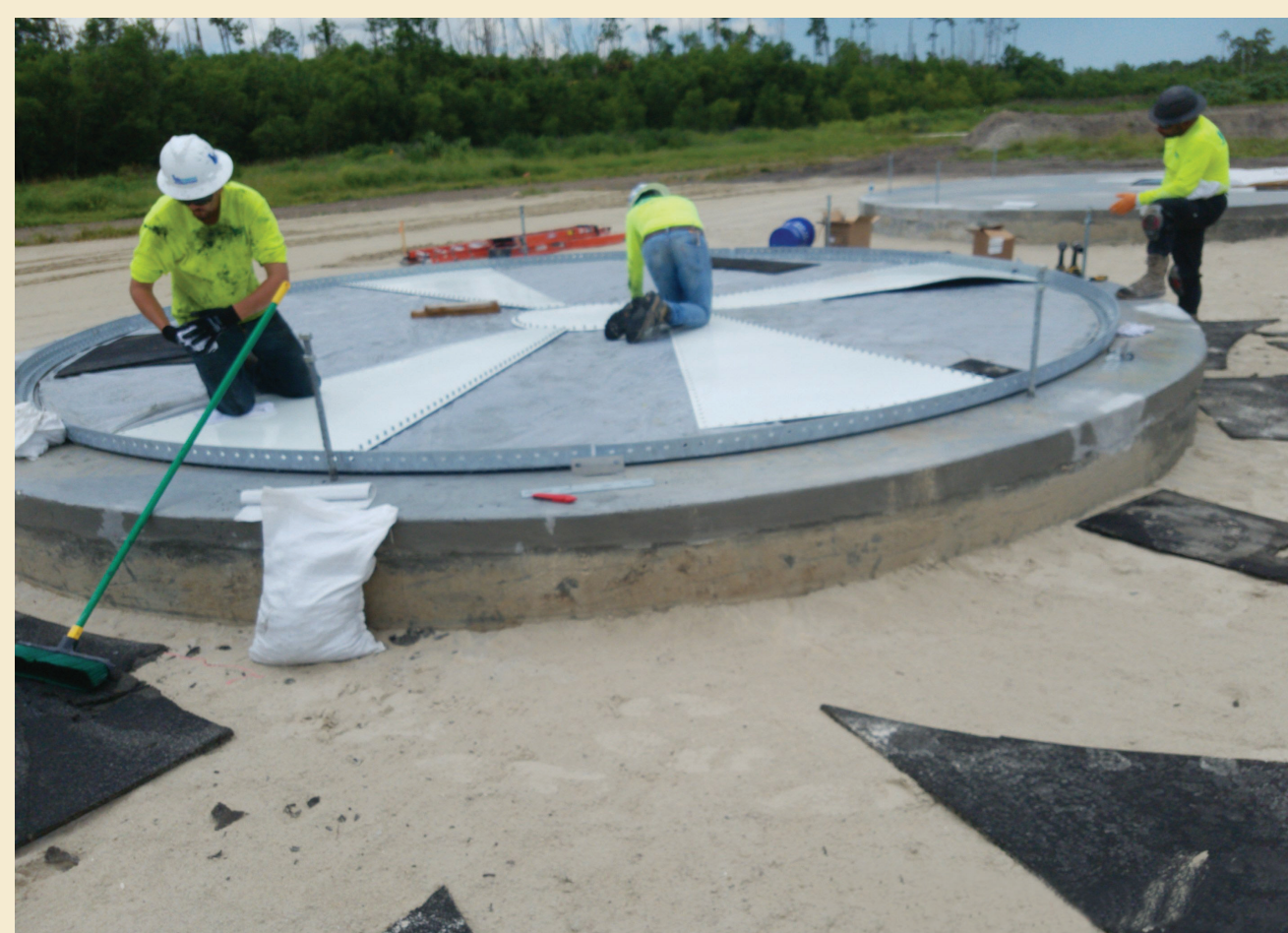
Aboveground Storage Tank Construction
