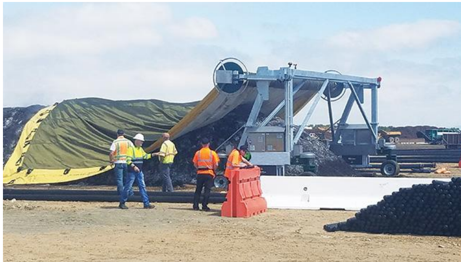
Large scale composting. Photos courtesy of SCS Engineers.
