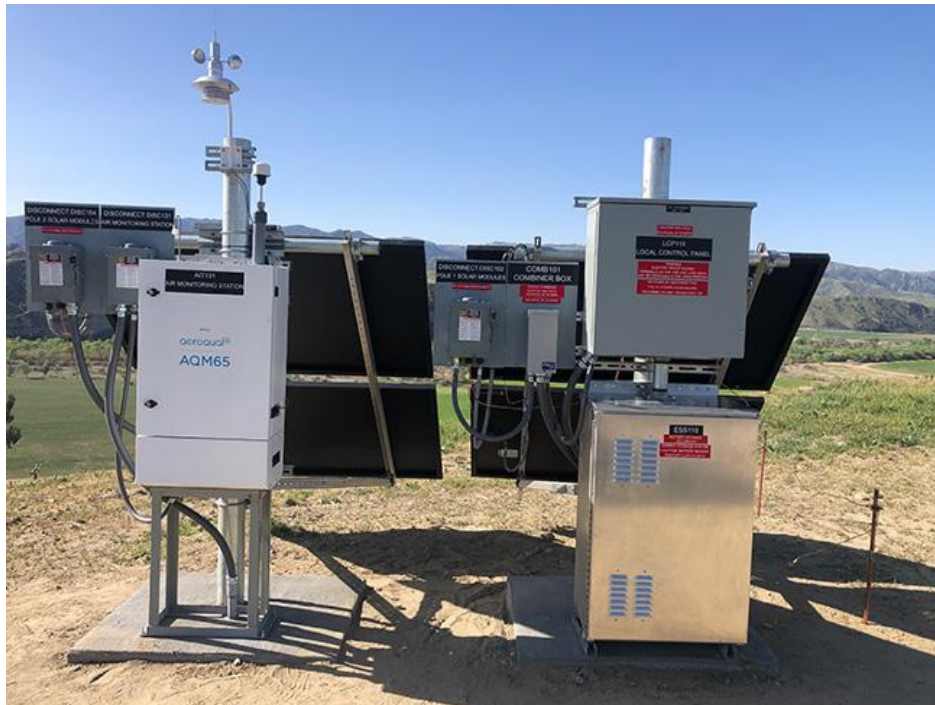
Air monitoring powered by renewable energy.
