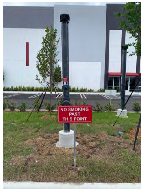
Passive Gas Vent Riser (typ.)
